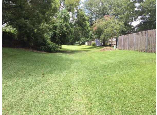
Picture 8D: Lateral 103 (Culverts 103-2 and 103-3) looking north from station 33+00. (Reference E-3.1)
