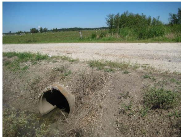
Picture 14E: Looking north at culvert 104-4 (Reference E-4.1)
