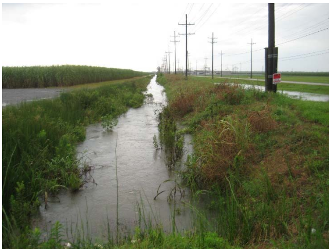
Picture 3E: Lateral 102 looking north from station 31+00 (9/26/2018 Rain Event) (Reference E-2.1)
