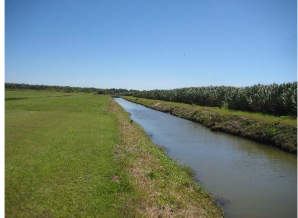
Picture 12F: Sub-lateral 103D Looking east from 520+00. (Reference E-3.4)
