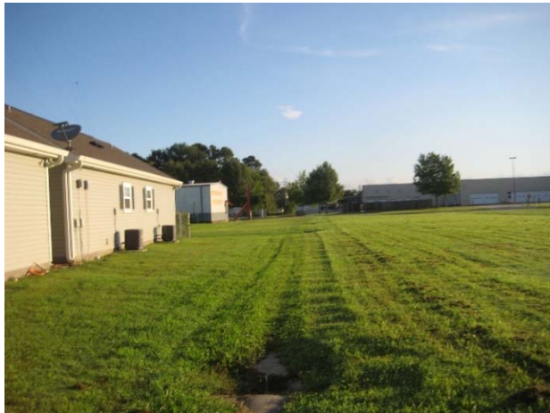
Picture 5A: Sub-lateral 102B looking north at culverted section from station 310+00. (Reference E-2.4)
