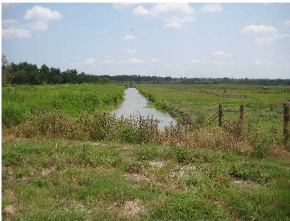
Picture 16A: Sub-lateral 104B looking east from station 14+50 (Reference E-4.1)
