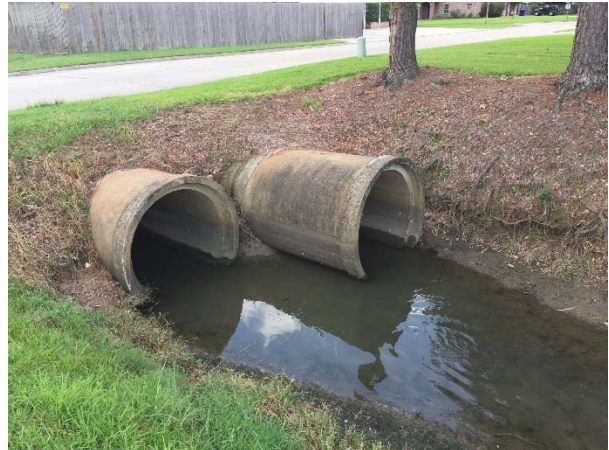
Picture 9F: Looking east at culvert 130A-5 (Reference E-3.1)
