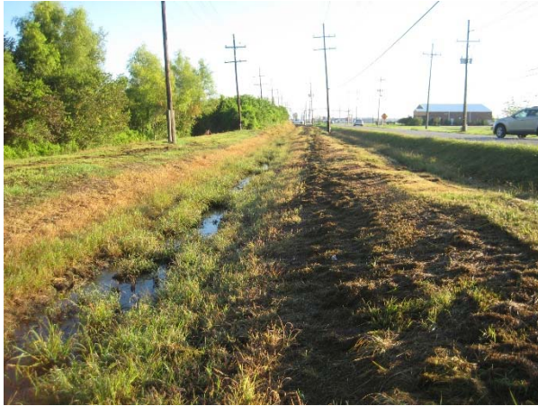
Picture 7C: Sub-lateral 102D Looking north from station 605+00 (Reference E-2.4)
