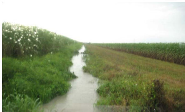
Picture 2A: Sub-Lateral 101A Looking north from station 216+00 (Reference E-1.1)
