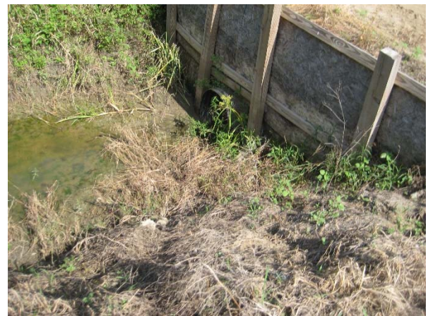
Picture 3B: Sub-Lateral 101B culvert crossing at station 11+50 (Reference E-1.2)
