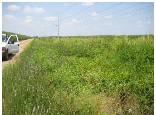
Picture 3F: Lateral 102 looking north from station 62+00 at sediment dams. (Reference E-2.2)
