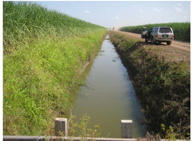
Picture 1F: Lateral 101 Looking south from station 62+00 (Reference E-1.2)
