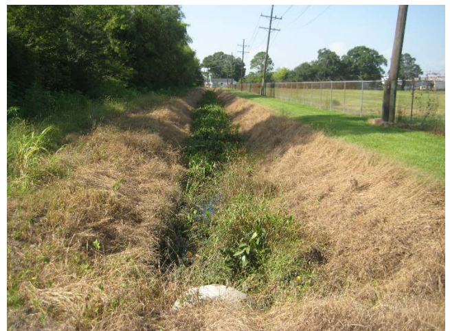
Picture 1B: Lateral 101 Looking south from station 8+00 (Reference E-1.1)
