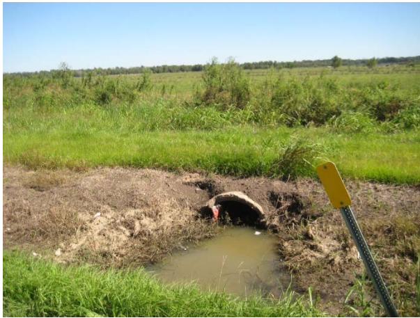
Picture 18A: Looking east at culvert 105A-2. (Reference E-4.1)
