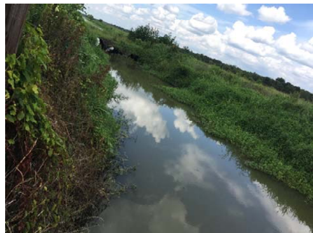
Picture 8F: Lateral 103 looking north from station 70+00. Culverts 103-4 within Lateral 103. (Reference E-3.2)
