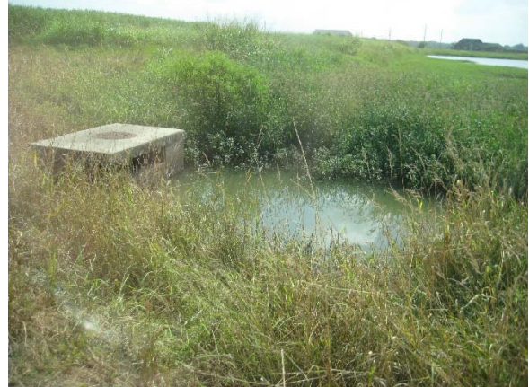
Picture 12B Concrete outfall structure 1 within regional detention pond. (Reference E-3.4)
