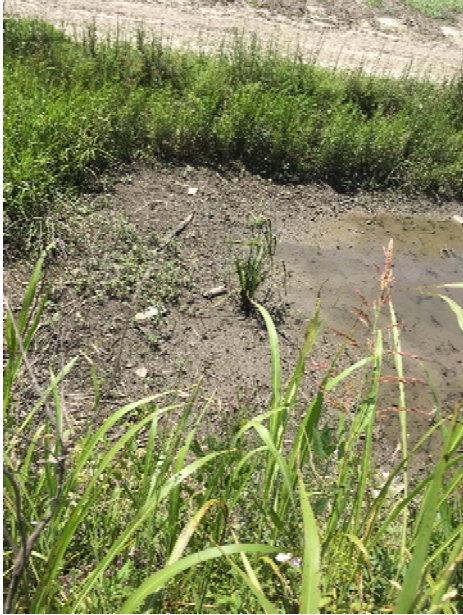
Picture 3G: Lateral 102 sediment dam near station 55+00 (Reference E-2.2)
