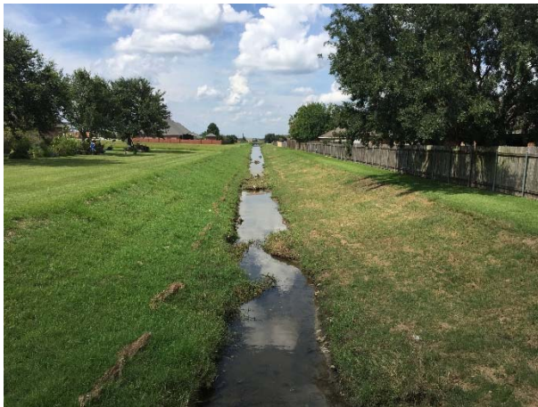
Picture 10A: Sub-lateral 103B looking north from station 300+50 (Reference E-3.4)
