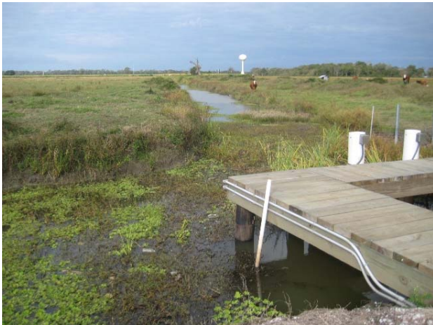
Picture 17E: Lateral 105 and city pump station looking west from station 158+00. Lateral 104 entering picture from left side. (Reference E-4.1)
