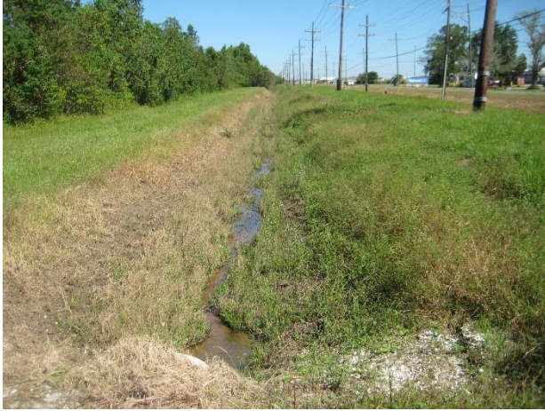
Picture 3C: Lateral 102 looking North from station 7+00 (Reference E-2.1)
