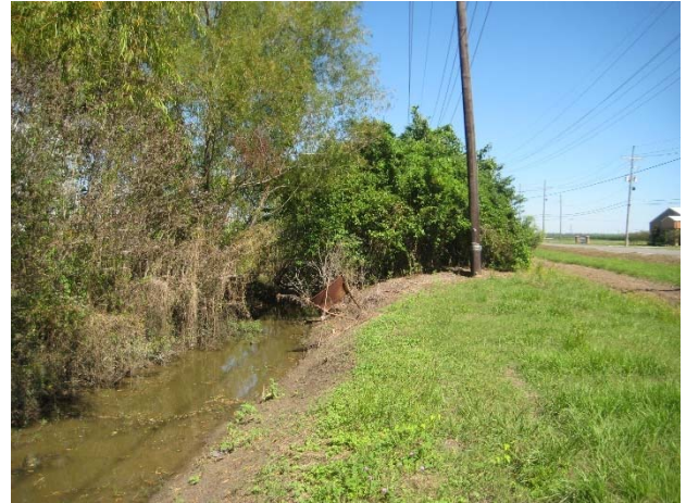
Picture 3D: Lateral 102 looking North from station 22+50 at the heavily vegetated ditch banks (Reference E-2.1)
