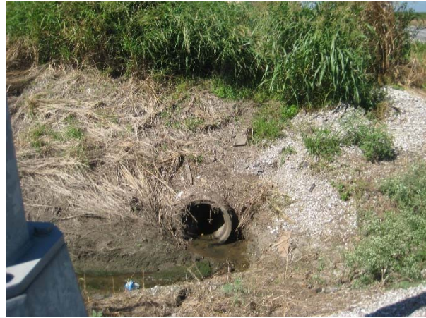
Picture 7D: Looking west at culvert 102D-2 (Reference E-2.4)
