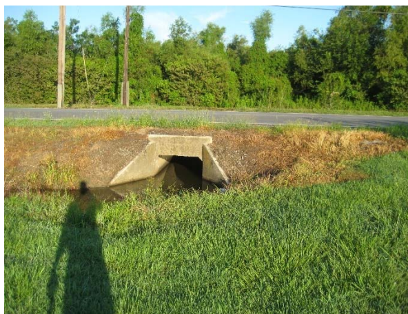
Picture 7B: Looking west at culvert 102D-1 (Reference E-2.4)
