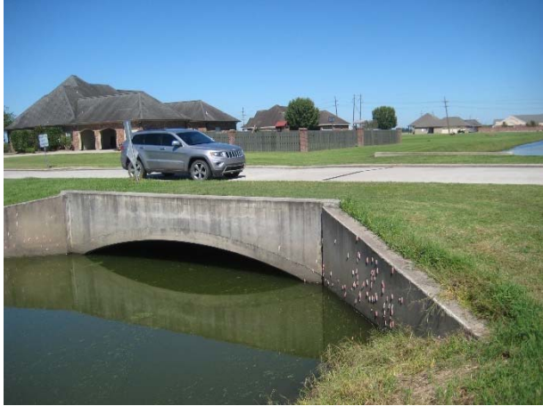
Picture 10E: Looking north at concrete bridge crossing 2 (Reference E-3.4)
