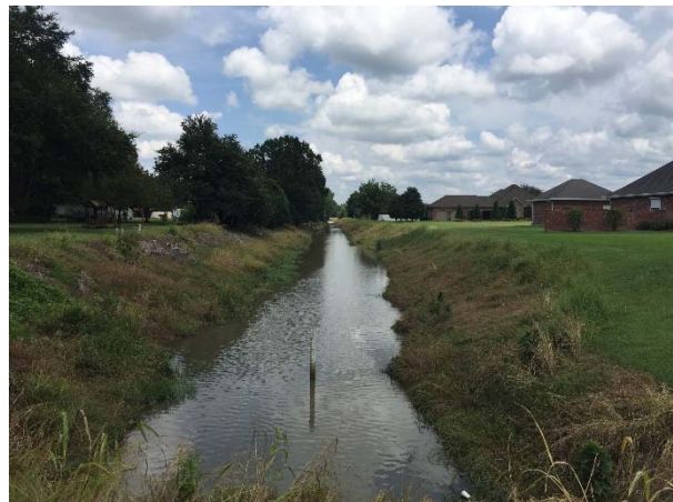
Picture 8B: Lateral 103 (Rienzi Canal) looking north from station 11+00 (Reference E-3.1)
