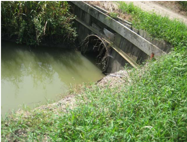
Picture 1E: Looking north at culvert 101-7 (Reference E-1.2)
