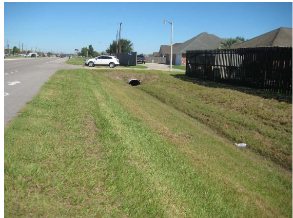
Picture 9B: Looking north at culvert 103A-2 (Reference E-3.4)
