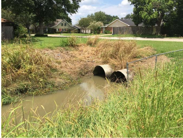
Picture 8C: Looking north at culverts 103-2 (Reference E-3.1)
