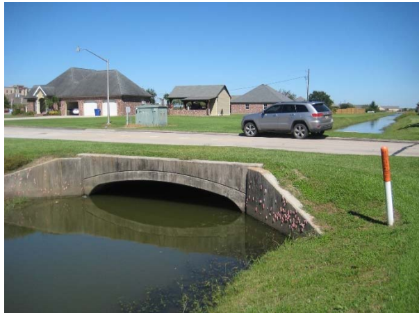
Picture 10C: Looking north at concrete bridge crossing 1 (Reference E-3.4)
