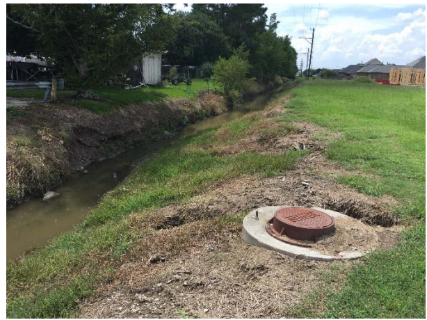
Picture 9H: Sub-lateral 103A Looking west from station 241+00 (Reference E-3.1)
