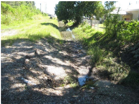
Picture 4C: Sub-lateral 102A looking east from station 506+00 (Reference E-2.1)
