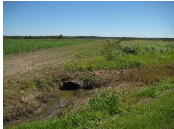
Picture 15B: Looking east at culvert 104A-2 (Reference E-4.1)
