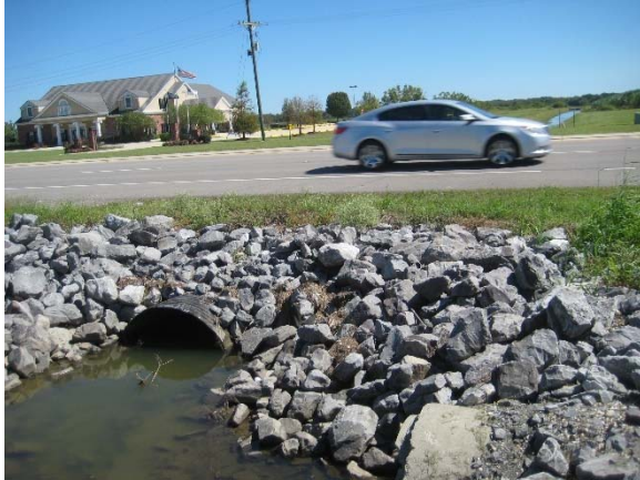
Picture 12E Looking east at culvert 103D-3 (Reference E-3.4)
