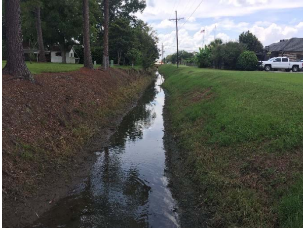
Picture 9E: Sub-lateral 103A Looking west from station 231+00 (Reference E-3.1)
