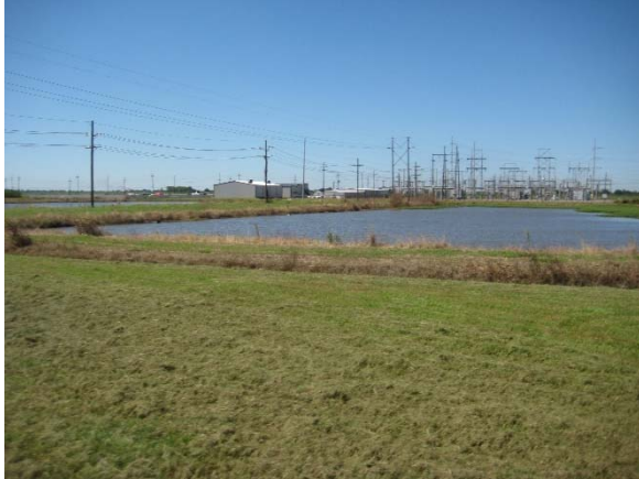
Picture 12A: Regional Detention Pond (Reference E-3.4)
