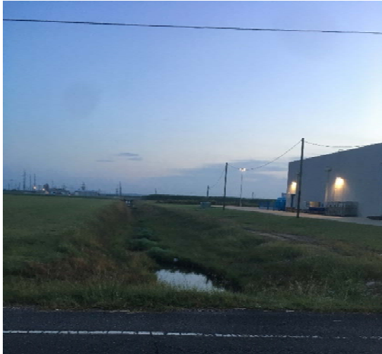
Picture 11C: Sub-lateral 103C looking north from station 408+00. Academy Sports on right hand side. (Reference E-3.4)
