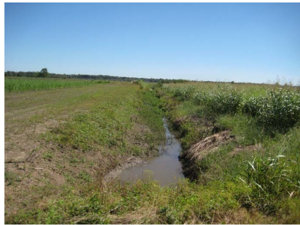
Picture 18B: Sub-lateral 105A looking north from station 402+00. (Reference E-4.1)
