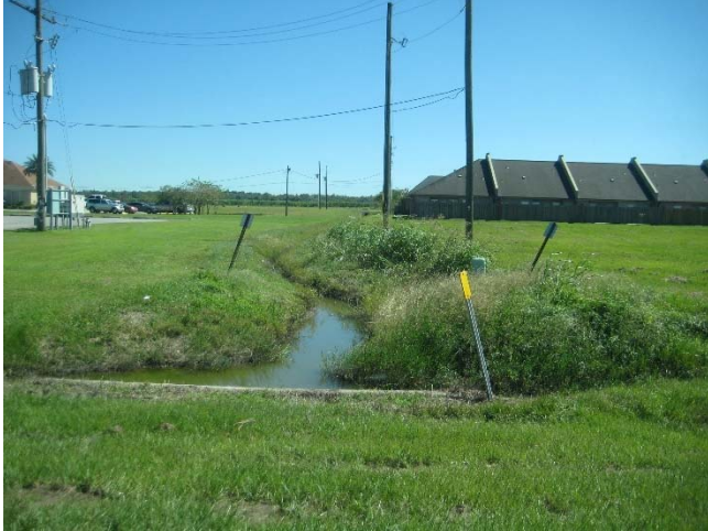
Picture 13C: Sub-lateral 103E looking east from North Canal Blvd at station 608+75. (Reference E-3.5)
