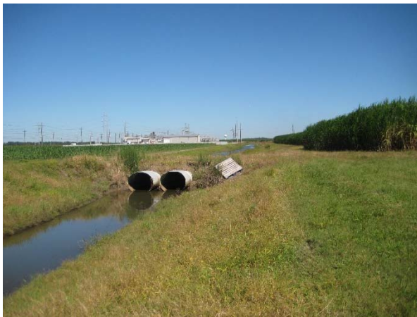
Picture 11E: looking north at culvert 103C-2 (Reference E-3.4)
