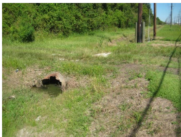
Picture 3A Looking North at culvert 102-1 (Reference E-2.1)
