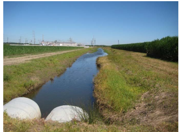
Picture 11F: Sub-lateral 103C looking north from station 415+00. Culvert 103C-2 in foreground. (Reference E-3.4)
