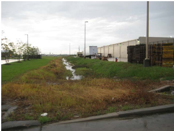
Picture 11A: Sub-lateral 103C looking north from station 400+00 @ Westover Drive (Reference E-3.4)
