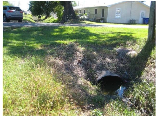
Picture 4B: Looking east at culvert 102A-1 (Reference E-2.1)
