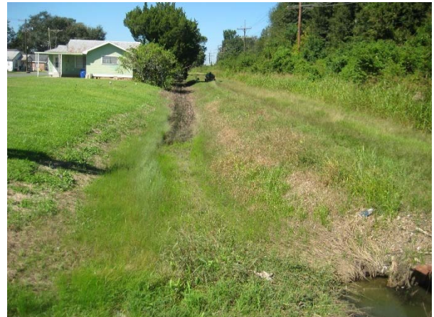
Picture 4D: Sub-lateral 102A looking west from station 511+00 (Reference E-2.1)
