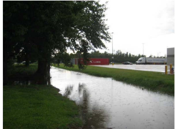
Picture 6B: Sub-Lateral 102C looking west from station 408+00 (Flooded Conditions) (9/26/2018 Rain Event) (Reference E-2.4)
