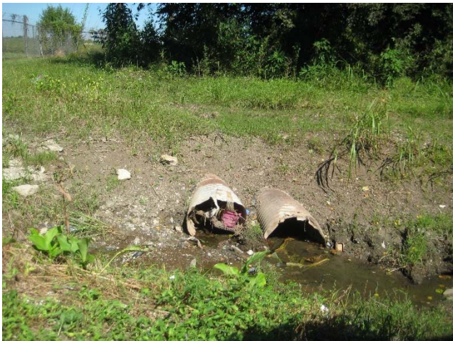
Picture 1A: Lateral 101 Looking north to culvert 101-1 (Reference E-1.1)
