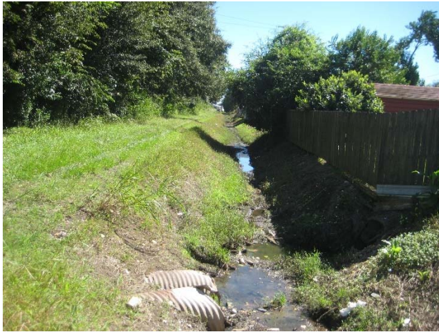
Picture 4A: Sub-lateral 102A looking east from station 500+00 (Reference E-2.1)
