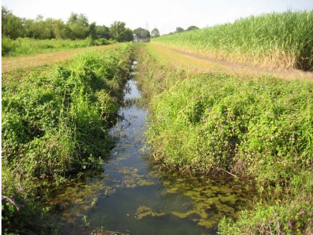
Picture 1C: Lateral 101 Looking south near station 15+00 (Reference E-1.1)
