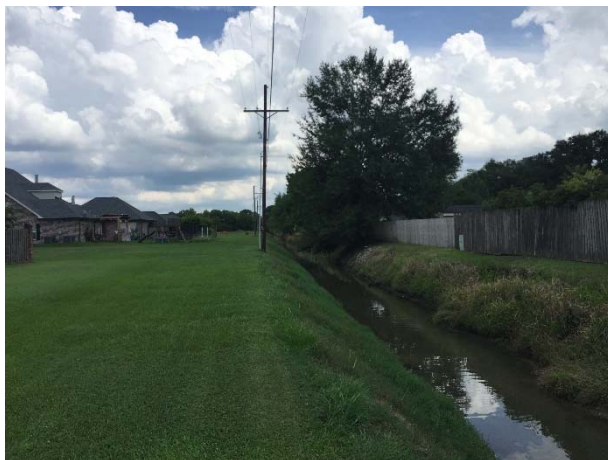
Picture 9G: Sub-lateral 103A Looking east from station 231+00 (Reference E-3.1)
