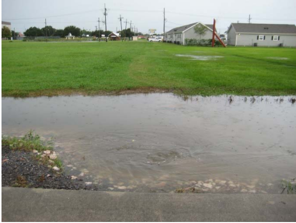
Picture 5E: Sub-lateral 102B looking south from station 312+50 (James Riviere St.) (9/26/2018 Rain Event) (Reference E-2.4)
