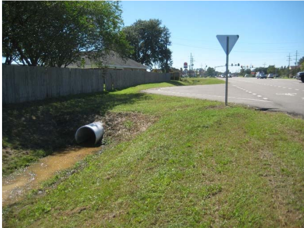
Picture 9A: Looking south at culvert 103A-1 (Reference E-3.4)
